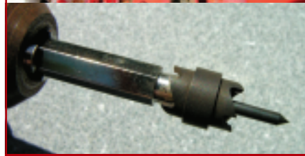
4. Some Early Bronco windshields seem to remove easily, but on this Bronco that chore was the hardest by far, and took hours. The first task is to carefully mark every spot weld exactly. On a bright sunny day I marked 90 welds. It was obvious that no robot welder made this Bronco. They were scattered everywhere in a random manner, and about 2/3 of all the welds were on the passenger side. Then you need to buy a special spot weld drill bit and carefully drill - circular saw really - every weld. These bits don't only cut through the first layer of hinge metal (and a little more), so if you center properly and get every weld, the old hinge a frame will pry right off. Mine wouldn't. A very careful inspection found five welds I missed, so they were drilled. Still couldn't break things loose. Using a socket under the hinge and repeatedly lifting and lowering the frame, it finally broke loose about five more welds that were so superficial they couldn't be seen and simply had to be broken free one at a time.
